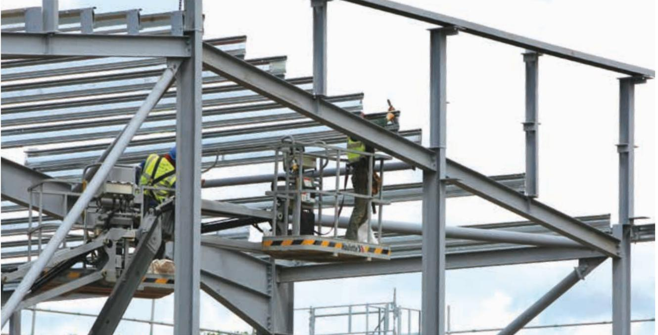
The Eaves Beam system incorporates a full range of cleats, brackets and struts providing solutions for all eave conditions. The economy and practicality of the Eaves Beam system complements Multibeam and Multichannel, providing a complete cladding support system.
