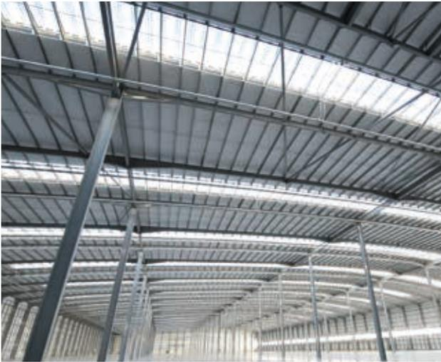
Multibeam purlins are suitable for all types of modern roof construction with bay sizes up to 15m.
