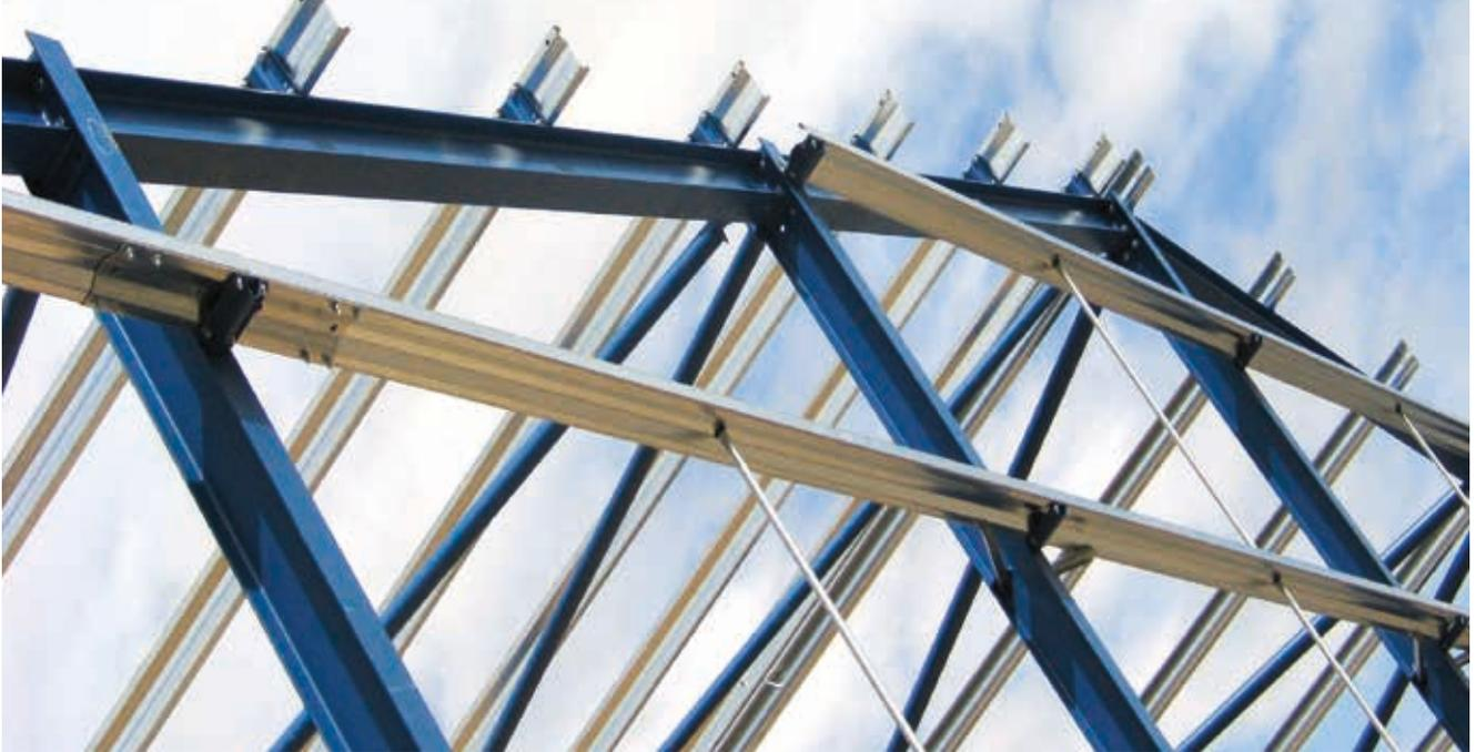
Multibeam cladding rail systems are suitable for all types of modern roof construction with bay sizes up to 15m and are designed specifically to support metal-clad walls in horizontal or vertical applications.
